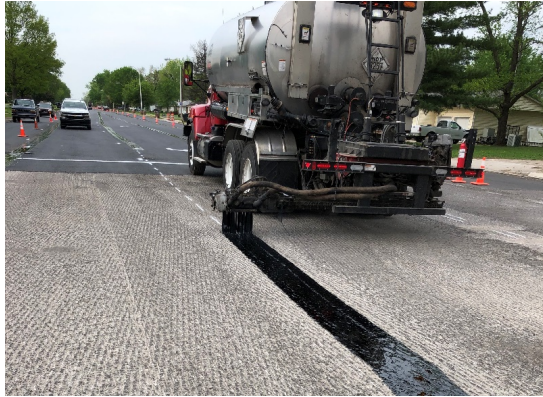
Figure 3 Heated pressure distributor and LJS spray bar
