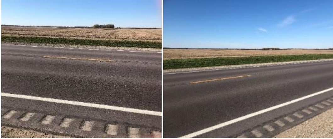
Figure 25. Control section on TH 22 north of the cemetery near 179th Street
