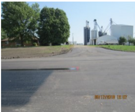
Figure 11. Start of J-Band section at farm driveway
