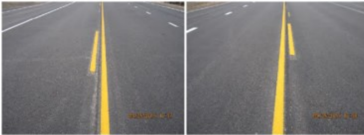
Figure 1 J-Band US169, Good condition.
