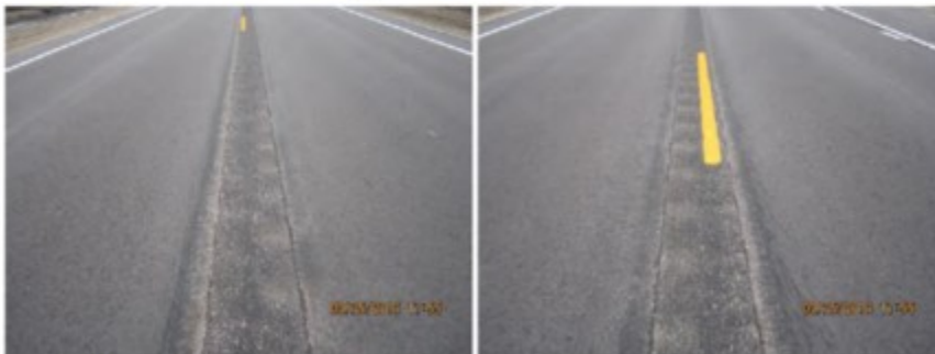
Figure 4 TH 22 J-Band. Good condition.
