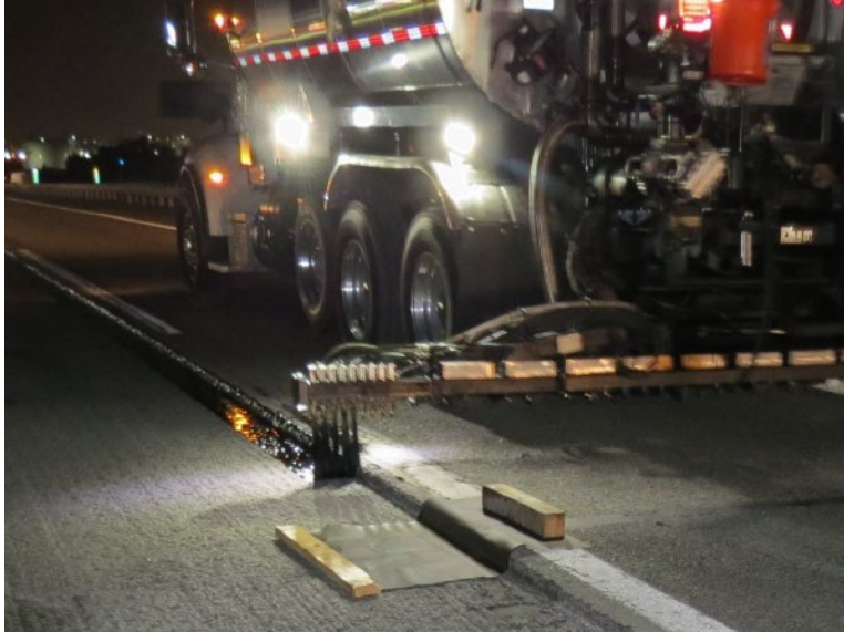
Figure 2 – New Jersey Turnpike Project (Also Showing Calibration of Application Rate)
