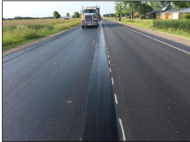
Figure 5: Application of tack coat material following VRAM along Illinois SR-1.
