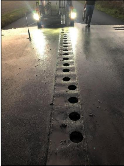
Figure 4: Example of coring along Lowell test section.
